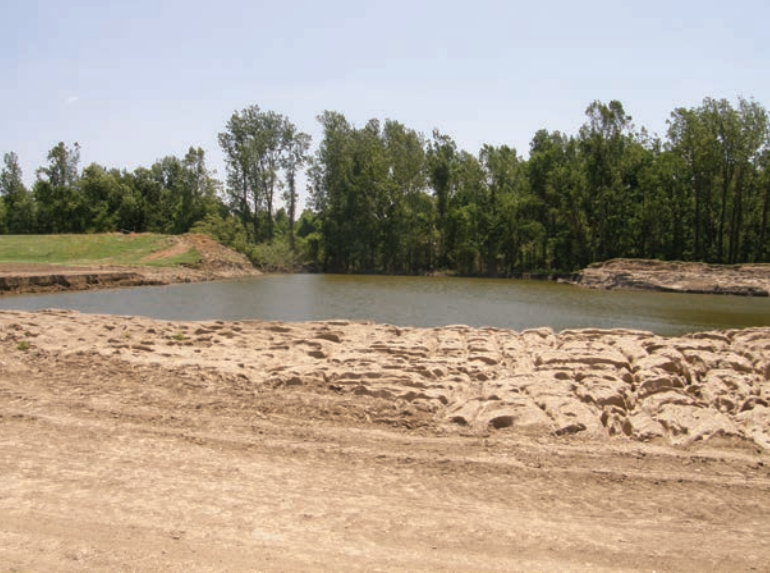
FIGURE 1.1 The Birds Point levee breach created a crater lake that extended many feet through the levee.
