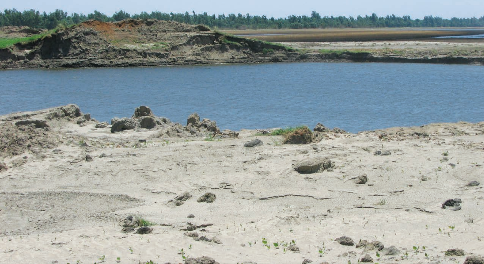
FIGURE 16.5 The Birds Point levee was the site of the first explosion on May 2, 2011, that opened the New Madrid Floodway and relieved river pressure on the Cairo floodwall. Remnants of the fuse plug levee and the crater lake extend into the adjacent agricultural lands.
