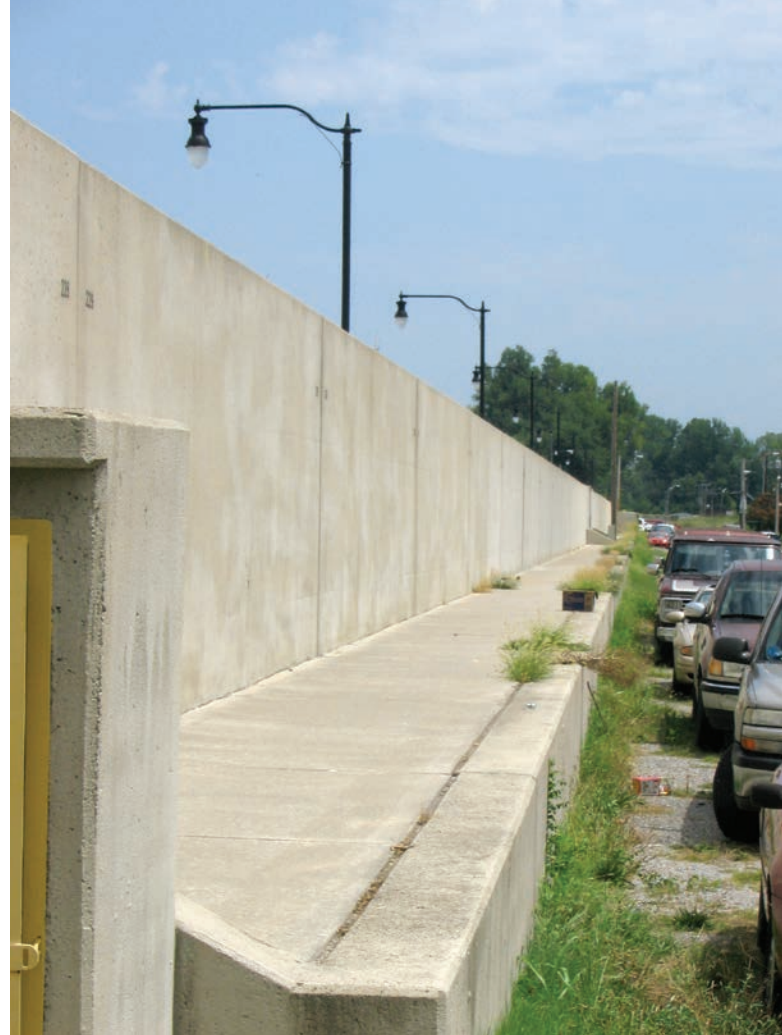
FIGURE 8.5 The concrete floodwall on the east side of Cairo, Illinois, protects the city from Ohio River flooding.
