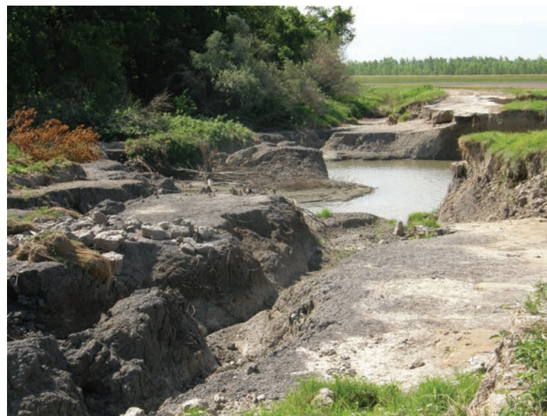
FIGURE 13.3 Gully development in the O'Bryan Ridge soybean field caused trees to fall into channels and undercut County Road 310.
