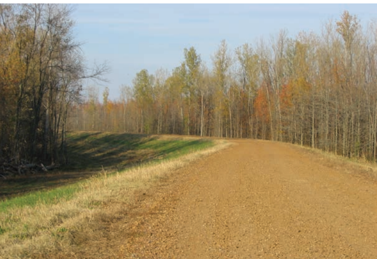
FIGURE 14.2 The diversion embankment redirects the middle Cache River water into the Mississippi River and blocks it from draining into the Ohio River via the lower Cache River.
