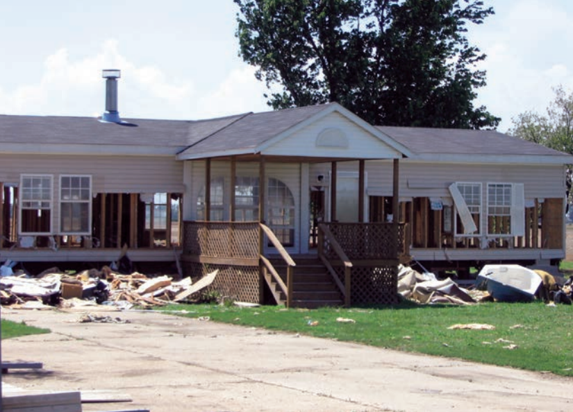
FIGURE 12.2 One of the 80 homes in the floodway damaged by the 6 to 10 feet of floodwater in 2011.
