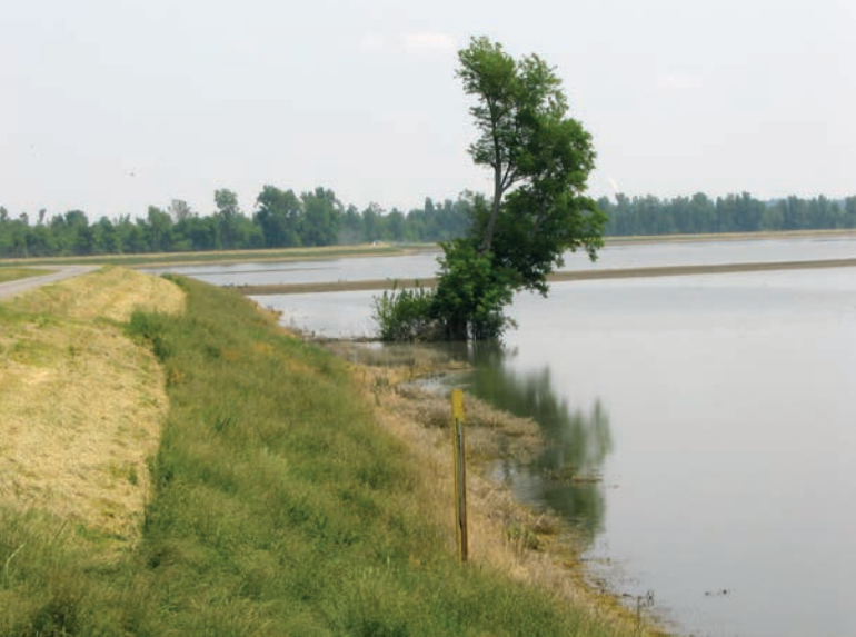
FIGURE 10.1 The New Madrid Floodway and basin still had four to six feet of floodwater on May 20, 2011, 18 days after the US Army Corps of Engineers induced a breach at Birds Point, Missouri.
