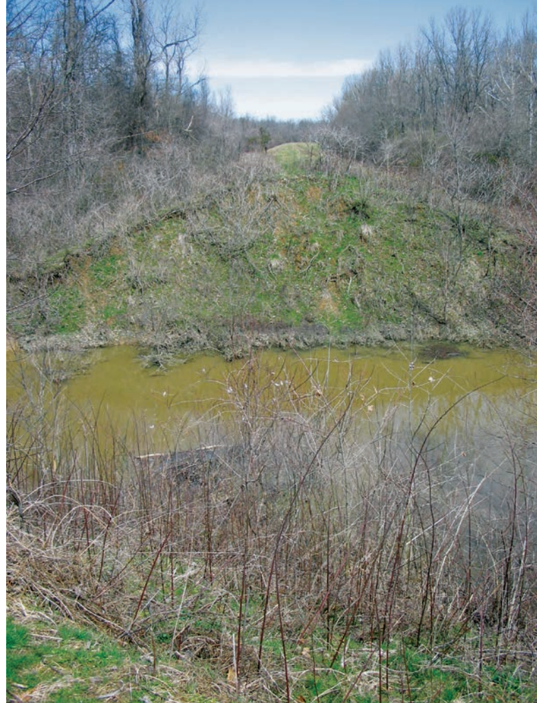
FIGURE 14.6 The unrepaired Karnak levee breach allows Cache River floodwaters to flow west toward the Mississippi River diversion.
