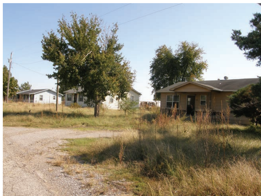
FIGURE 12.5 Homes in the village of Pinhook in November of 2011 were abandoned after they were damaged by 6 to 10 feet of floodwater.
