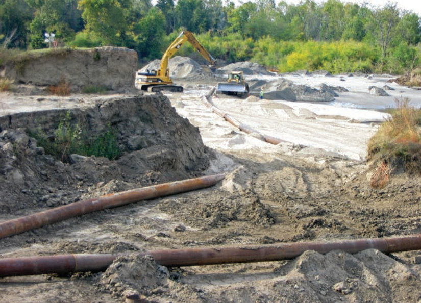
FIGURE 11.1 The Big Oak Tree levee blast site was repaired in October of 2011 and reconnected to the 62.5-foot frontline levee.
