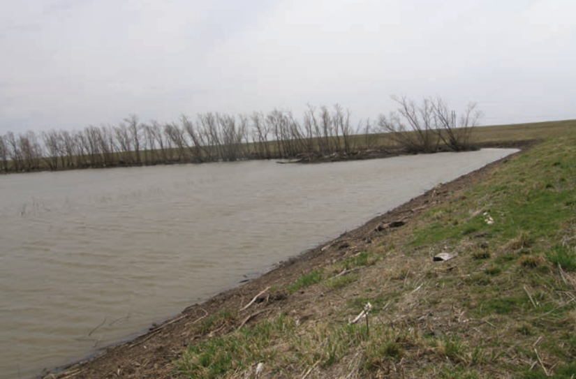
FIGURE 4.7 The Pigeon Creek settling basin west of Hull, Illinois, is currently active during high runoff and flooding.
