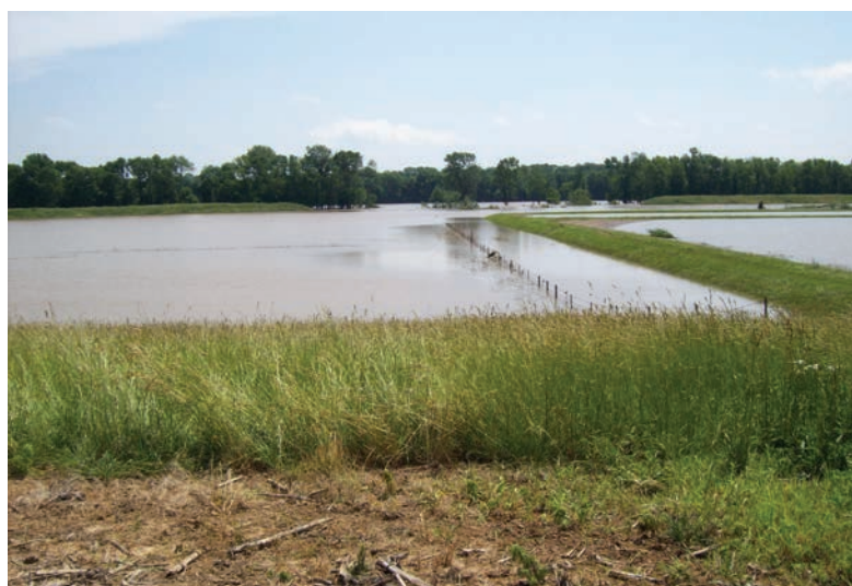
FIGURE 9.3 Full temporary storage ponds surrounded by flooding from the Embarras River near Sainte Marie, Illinois, in June of 2008. Photo credit: Ken Flexter, Jasper County Natural Resources Conservation Service Field Office, Newton, Illinois.
