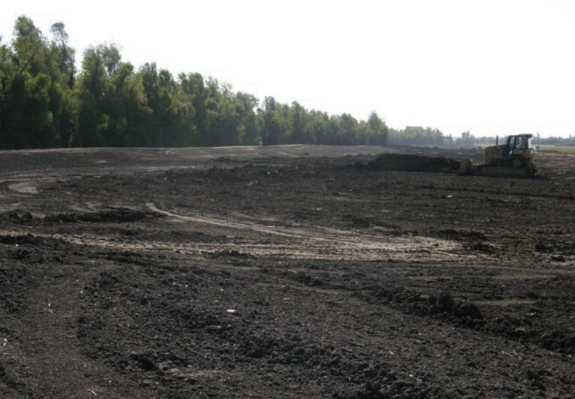
FIGURE 8.4 A levee at Birds Point, Missouri, is reconstructed after the induced breach of 2011.
