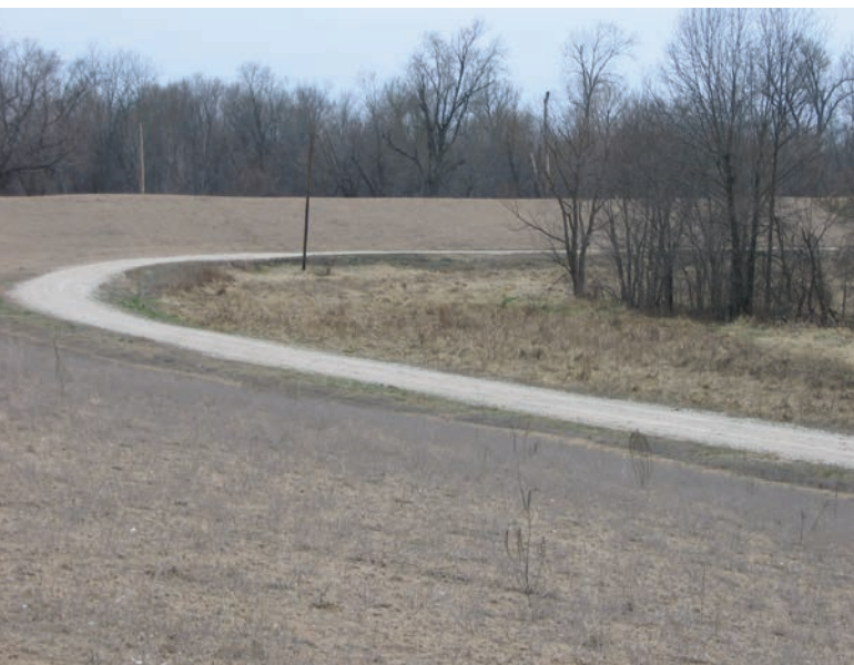
FIGURE 4.6 The merged Mississippi River and Kiser Creek Diversion levee blocks the Sny River channel flow, and water has to be pumped over the levee to the Mississippi River.
