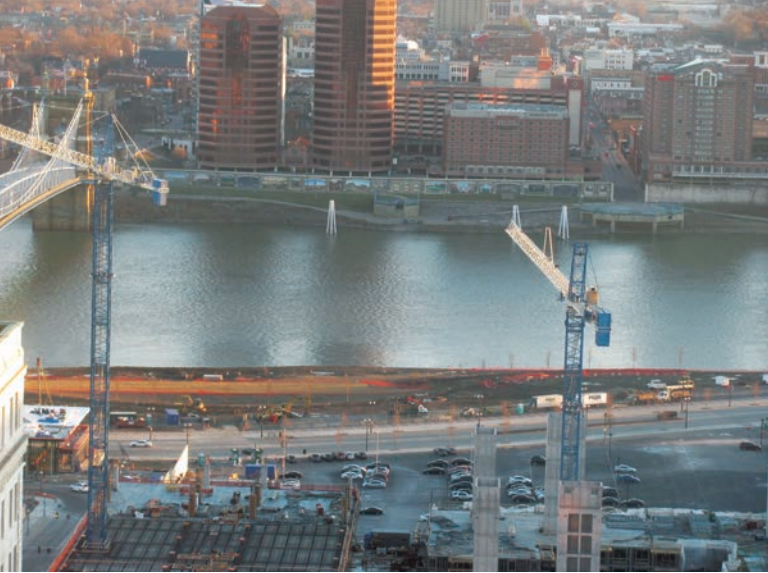
FIGURE 18.8 The Covington to Cincinnati bridge was the only functioning bridge crossing from Steubenville, Ohio, to Cairo, Illinois, during the 1937 flood.
