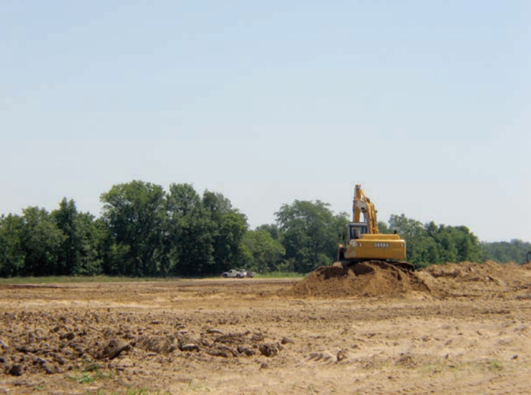
FIGURE 9.7 Sand is piled for transport off the agricultural lands previously protected by a levee.
