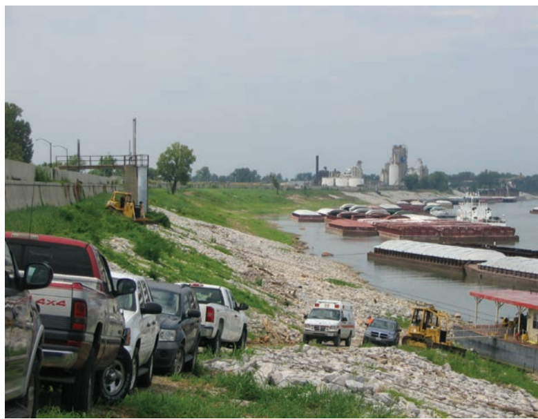
FIGURE 17.4 More than 64 feet of the Ohio River floodwall in August of 2012 were exposed when the Ohio River was at 12 feet during the drought. This was 50 feet lower than the May 2, 2011, high water mark.
