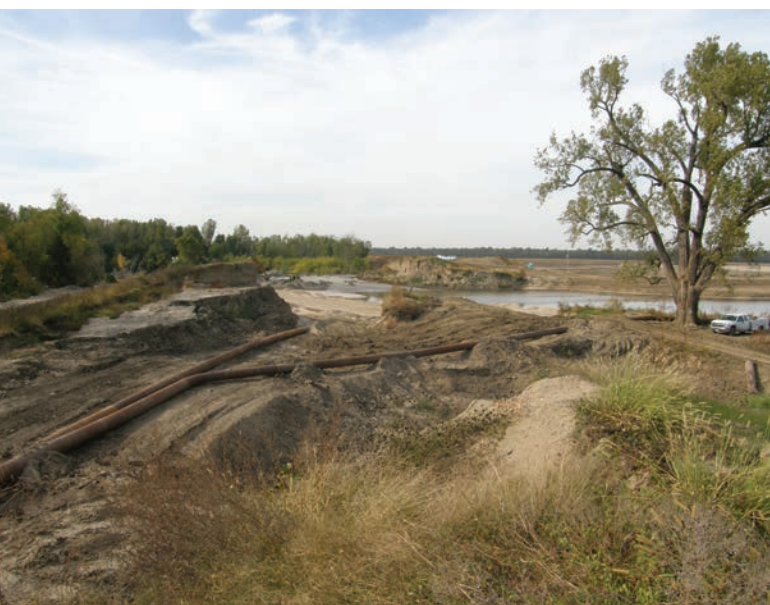
FIGURE 10.6 A crater lake was formed at the Big Oak Tree frontline levee when the fuse plug was blown and floodwaters rushed into the floodway.
