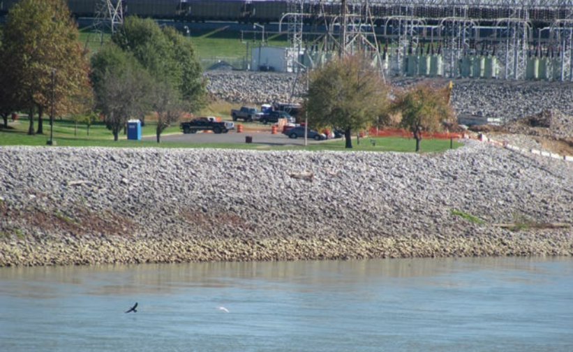
FIGURE 20.3 The Barkley Dam generates hydroelectric power for the region.
