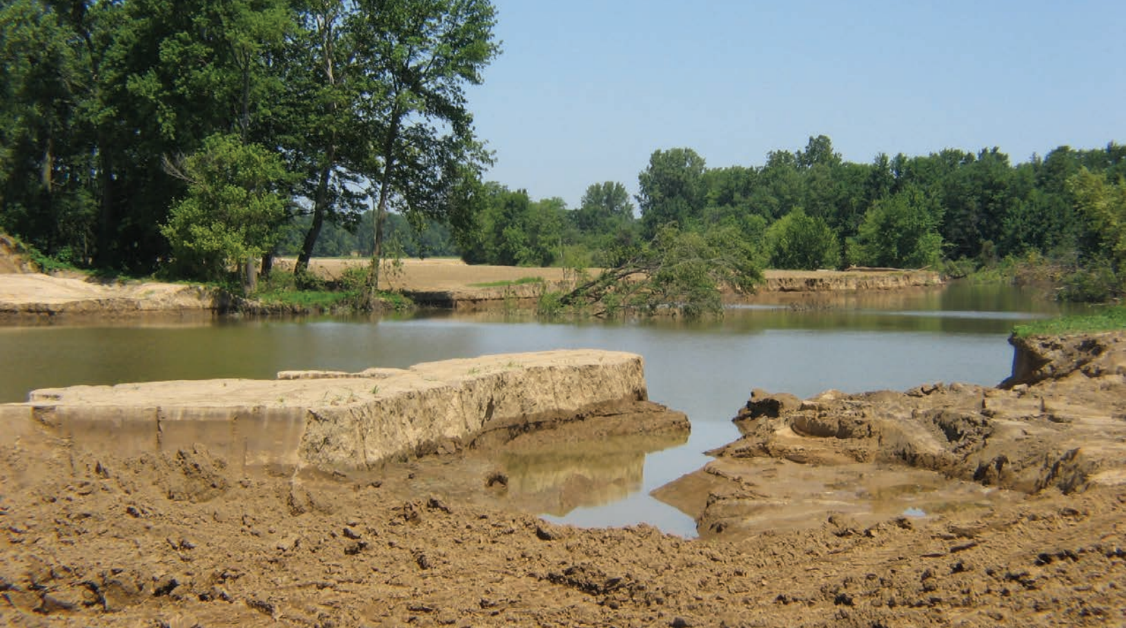
FIGURE 9.5 In the background is the Embarras River, Illinois, adjacent to a missing 300-foot section of the levee and the crater lake that was created by rushing waters.
