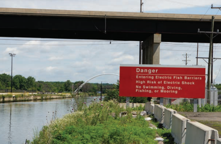
FIGURE 23.4 Electric fish barriers constructed in the Chicago Sanitary and Ship Canal are designed to prevent invasive species of Asian carp from passing from the canal into Lake Michigan.
