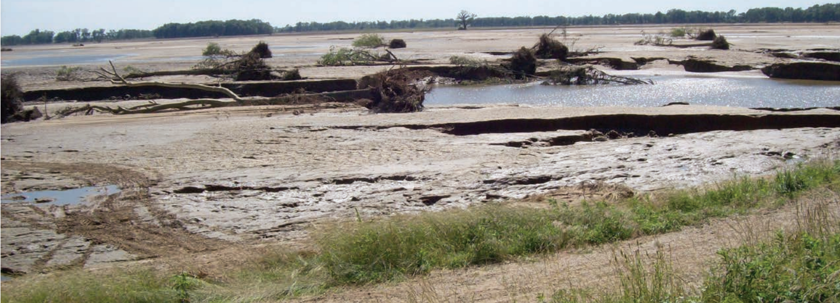
FIGURE 8.11 Trees on the river side of a levee are transported by floodwaters through the levee breach into adjacent fields.
