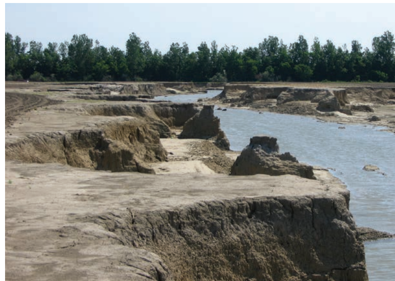
FIGURE 8.8 An O'Bryan Ridge gully created from an induced breach in May of 2011 is filled with water and removed land from agricultural production.
