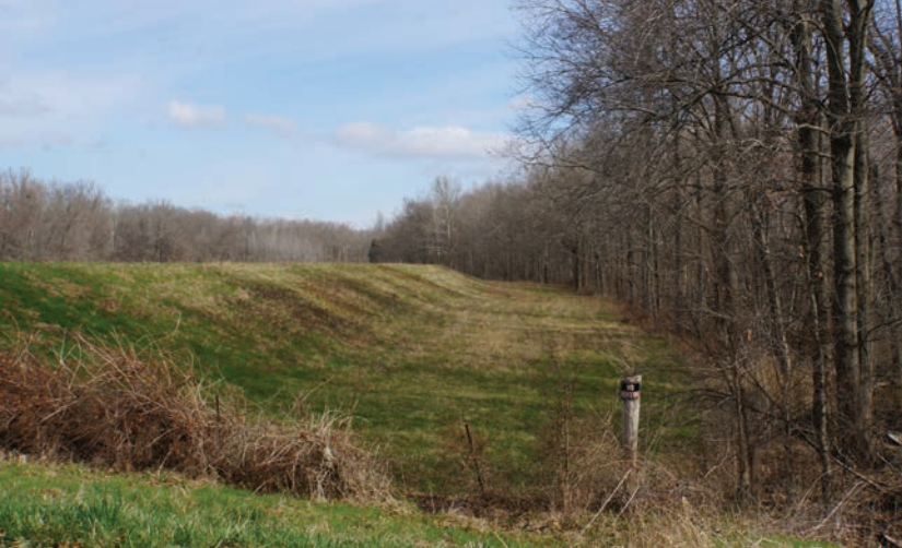
FIGURE 14.5 The Reevesville levee protects the Main Ditch from Bay Creek floodwaters.
