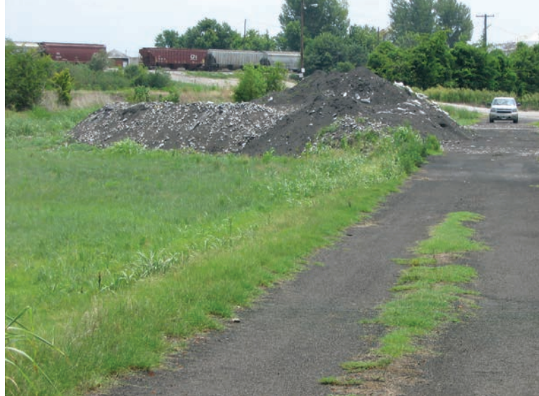
FIGURE 17.3 The raised railroad bed is visible in the background of the 40th Street mega sand boil in Cairo near the water treatment plant. The mega sand boil was filled in and covered with a 13.2-foot-high pile of fly ash cinders.
