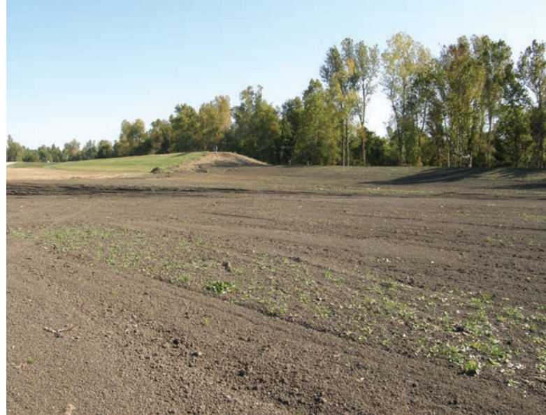
FIGURE 11.2 The 2011 Birds Point levee patch built to 51 feet rather than the original 60.5 feet.
