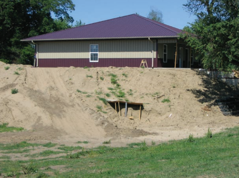
FIGURE 12.4 One of the new homes was built on 10 feet of soil materials to prevent future flood damage.
