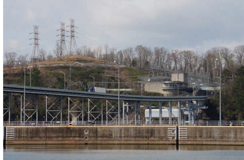
FIGURE 19.8 Watts Bar Dam on the Tennessee River between Knoxville and Chattanooga, Tennessee, generates hydroelectricity, contributes to downstream flood management, and enables navigation on the Tennessee River via its locking system.
