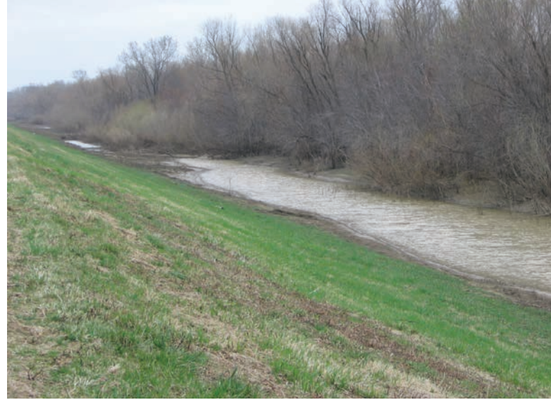
FIGURE 4.4 The wide Kiser Creek Diversion channel is timberland between the two levees just before it drains into the Mississippi River.
