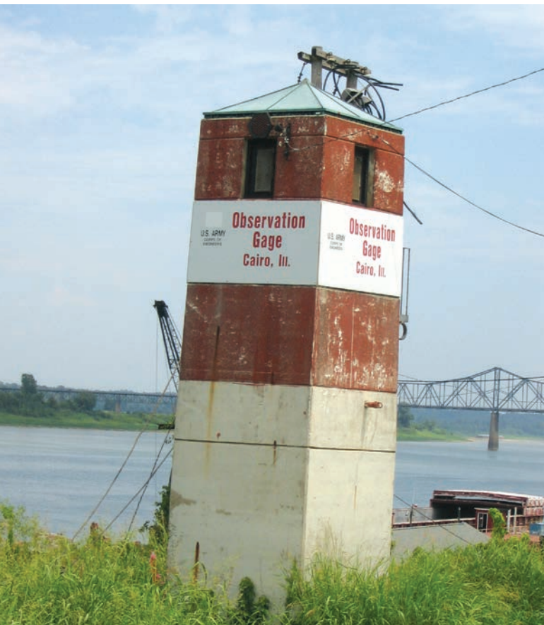
FIGURE 1.2 The Cairo, Illinois, river gage on the Ohio River is used to determine river height and when it is necessary to open the Birds Point-New Madrid Floodway to relieve downstream river pressure.
