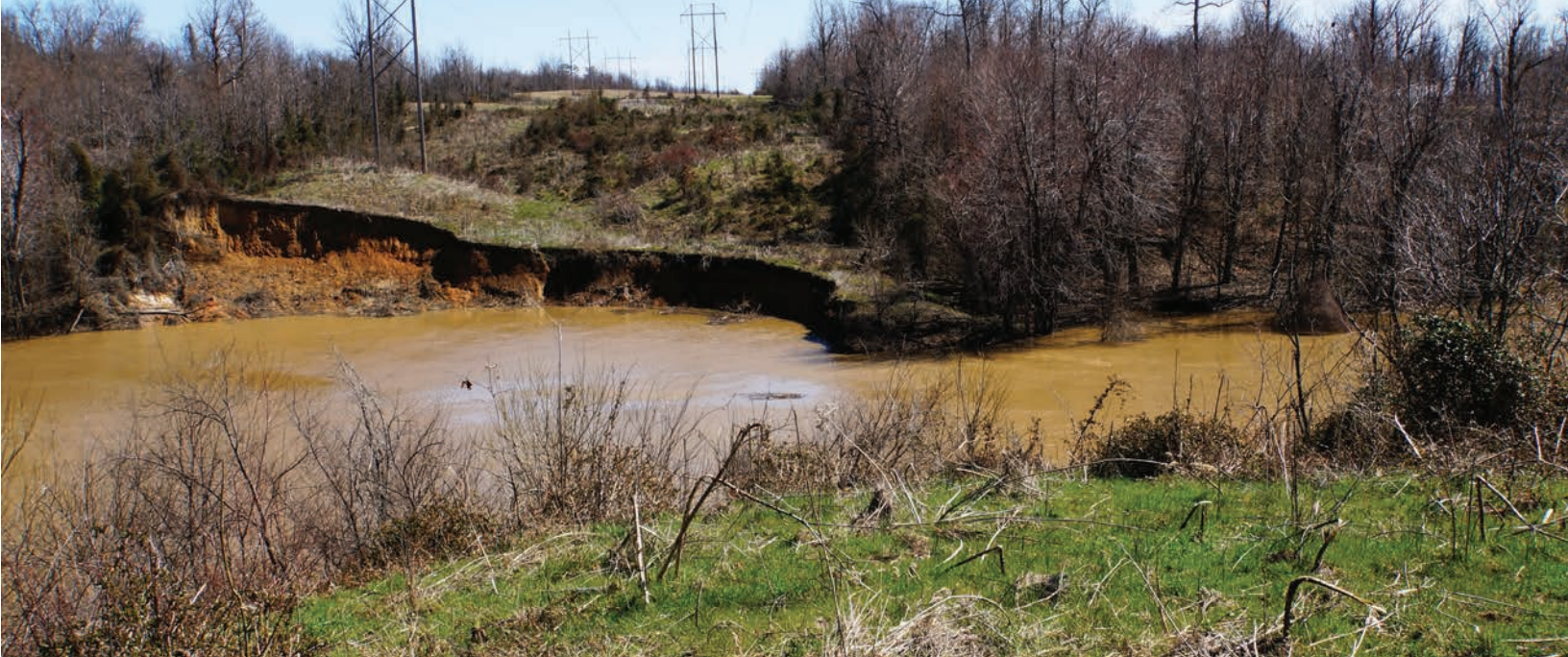
FIGURE 14.3 The Post Creek Cutoff dug in 1912 has highly eroded banks and sediment loads that are deposited at its mouth as it drains into the Ohio River.
