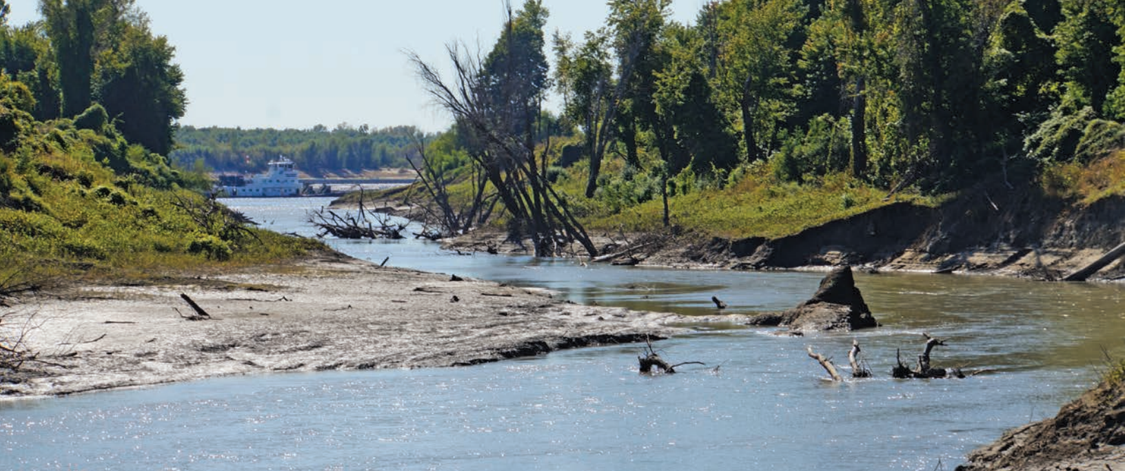
FIGURE 7.1 A riverboat on the Mississippi River can be seen passing the outlet of Main Ditch that drains through the 1,500-foot frontline levee gap at New Madrid, Missouri, to the Mississippi River.
