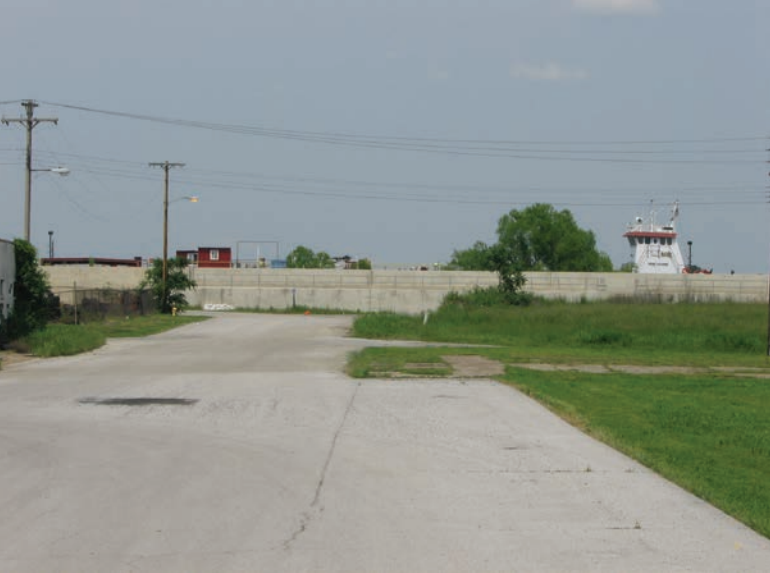
FIGURE 16.1 The Cairo floodwall is built on the Ohio River side at the bend in the river where an earthen levee would be difficult to maintain. With the river 10 feet above flood stage, a tugboat is visible behind the floodwall.
