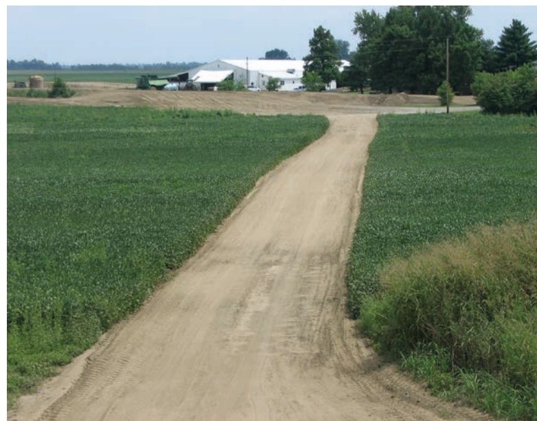
FIGURE 15.5 Post-2011 Len Small levee breach, many farmers built small levees around their farmsteads to protect against internal flooding and future breaching.
