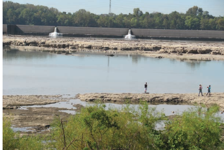
FIGURE 18.5 The McAlpine Dam at Louisville, Kentucky, and Clarksville, Indiana, controls water levels on the Ohio River and allows barges and boats to bypass the falls of Ohio (in the foreground). The dam, an elongated “Z,” protects the ancient fossil beds of the falls of Ohio and has “castellations” or waterfalls in the dam to ensure water reaches the wetland next to the dam even in dry months so as to maintain wetland plant and animal species.
