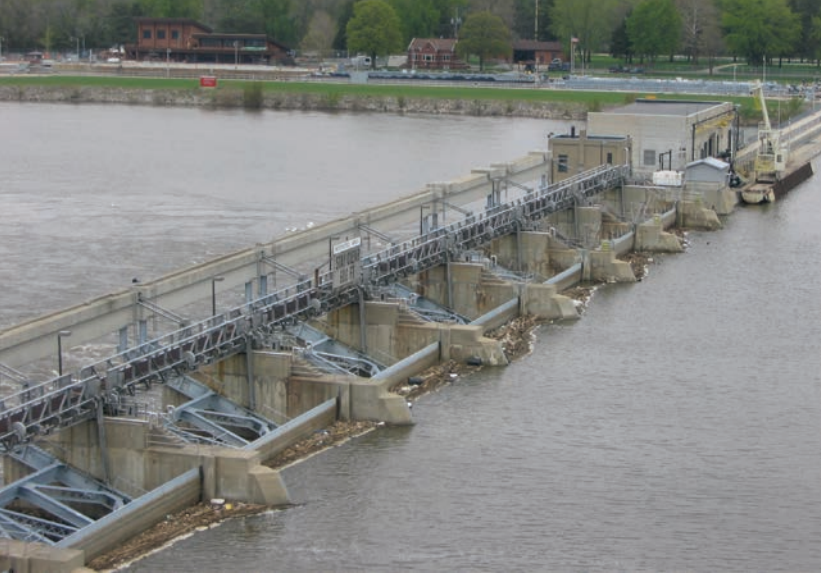
FIGURE 3.1 Starved Rock locks and dam help maintain the nine-foot navigation channel on the Illinois River waterway.
