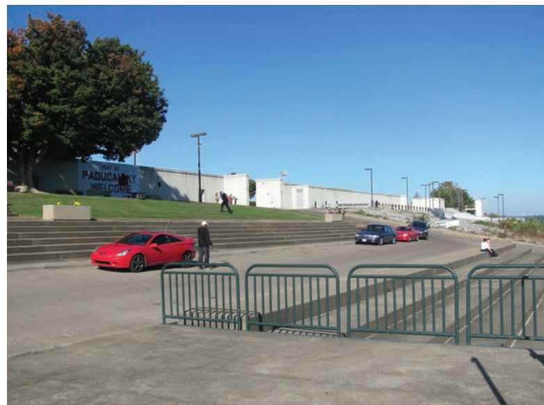
FIGURE 19.2 The river side of the floodwall at Paducah, Kentucky, is a park to view the Ohio River at low water and a protection against the river at high water. The floodwall was constructed after the 1937 flood, which destroyed most of downtown Paducah.
