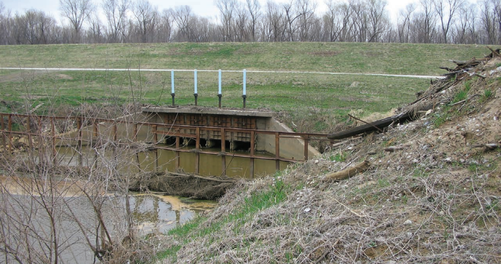
FIGURE 4.5 The Sny River aqueduct passes under the Kiser Creek Diversion channel.
