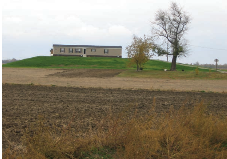
FIGURE 11.9 A home is rebuilt on an eight-foot-high mound of soils to protect against future flooding.
