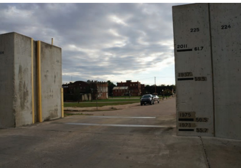
FIGURE 16.2 An open floodwall gate in Cairo shows city buildings and industries adjacent to the protective wall. The wall has never been breached, and high water crests since 1937 are marked to show the Ohio River height as recorded on the Cairo gage.
