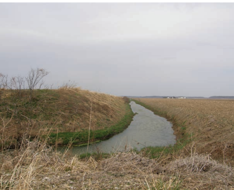
FIGURE 4.2 A 640-acre settling basin (McCraney) filled with sediments in the 1950s and is 7 to 10 feet above the bottomlands and 9 to 14 feet above the current drainage ditch.
