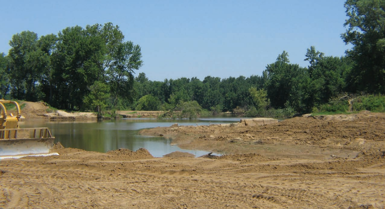
FIGURE 8.7 A crater lake extends 300 feet through the levee breach.
