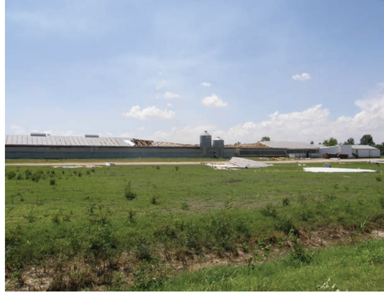
FIGURE 12.3 Farm structures including a hog confinement facility were damaged by floodwaters and wind when the floodway was opened in 2011.
