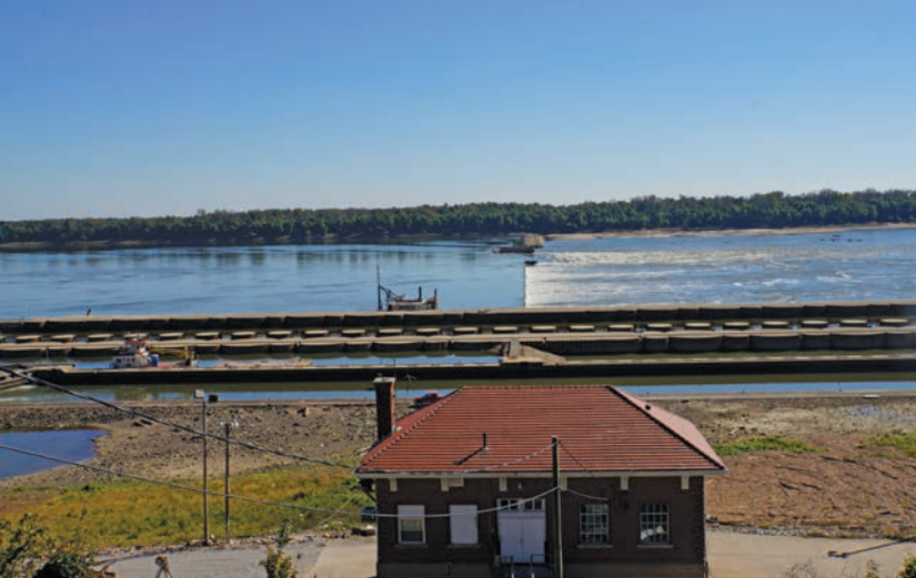
FIGURE 18.4 Lock and Dam 53 at 962 river miles downstream from Pittsburgh has an upper pool above the dam that extends about 23 miles to Lock and Dam 52.
